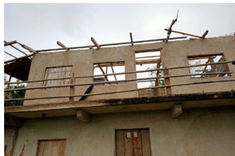
A house stripped of its roof sheet in Sierra Norte de Puebla, Mexico.
